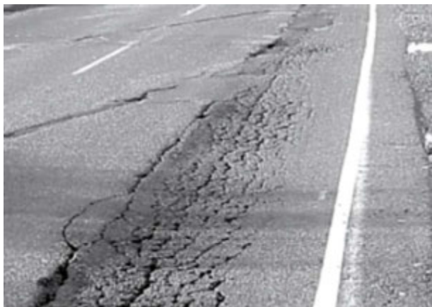
Figure 3.2: Pavement rutting: longitudinal vertical deformation of a pavement surface in a wheelpath
