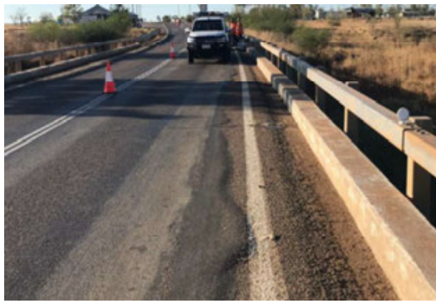
Figure 3.3: Pavement shoving: Lateral displacement of pavement structure by braking, accelerating or turning vehicles
