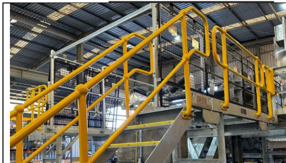
Handrail and Stair Treads
