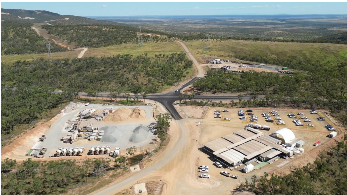
Figure 2 Destruction of open eucalyptus forests by a small part of the Clarke Creek wind farm - concrete batching part on the left, temporary offices on the right, and haulage roads for wind turbines climb the hills on the left after crossing HV transmission.
