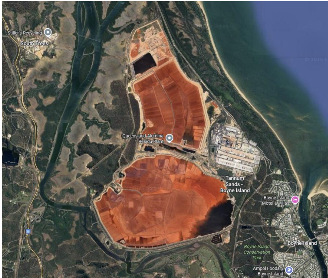
Figure 8 Qld Alumina red mud waste dump just to the south of Gladstone
