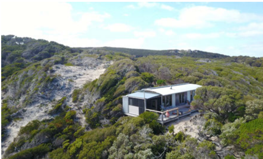
Figure 10 — The same building system delivered to a remote coastal site. Approximately 250 such dwellings have been delivered across Australia and overseas over twenty-five years, many in off-grid and very remote locations. Author's project; the interest is declared.
