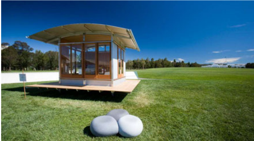
Figure 9 — A ReThink Prefab pod dwelling on the lawns at Old Parliament House, Canberra. Flat-packed into standard shipping containers, assembled by a small crew with hand tools on disturbance-free footings. Author's project; the interest is declared.
