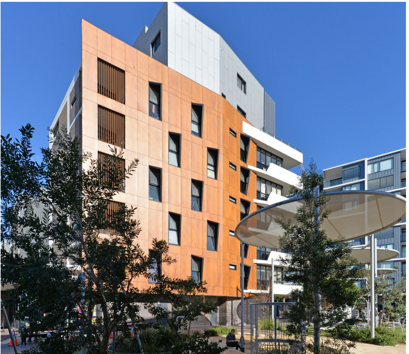
City West Affordable Housing, Green Square
