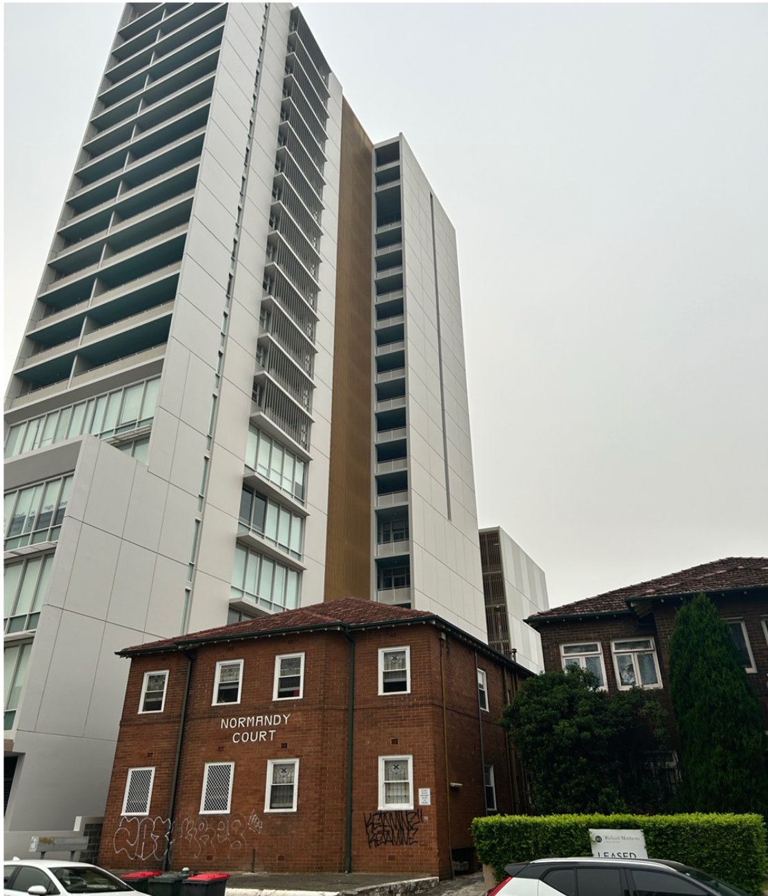
Figure 1: Site in Railway Parade Burwood NSW where a 2 storey apartment building persists despite a much larger upzoning. (source: Peter Phibbs)
