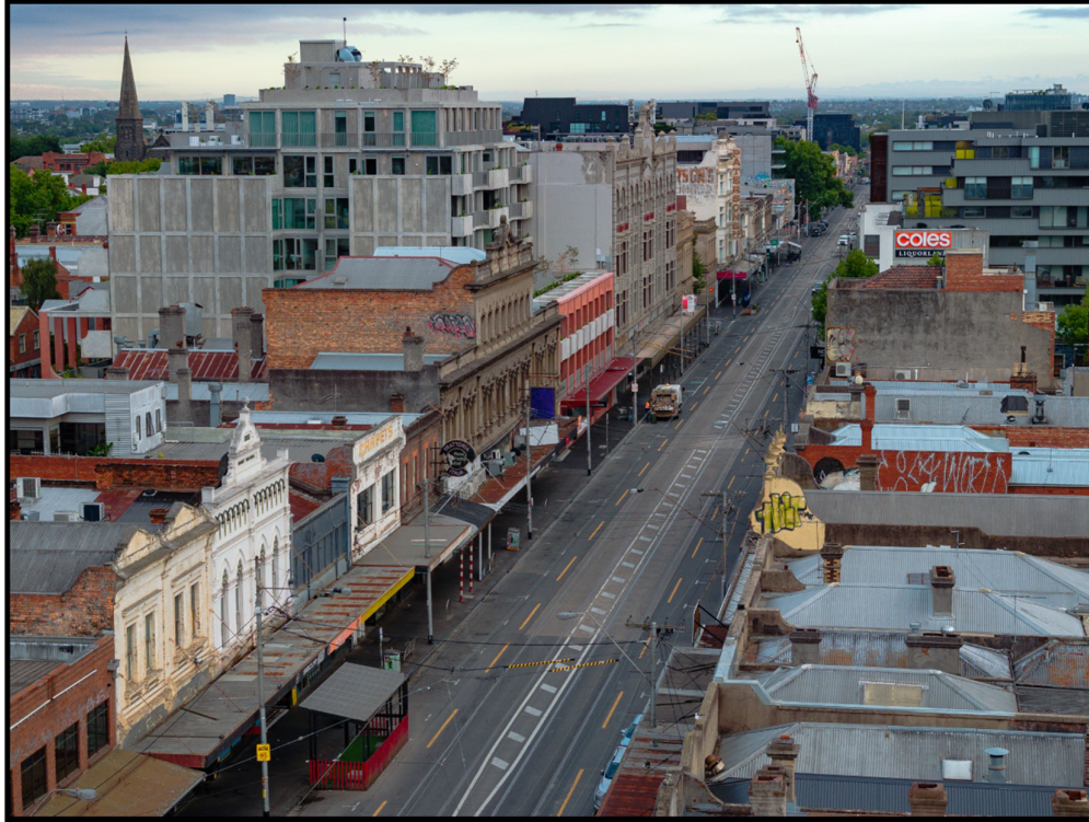
Development (residential and commercial) within a heritage precinct and Major Activity Centre Smith Street, Collingwood 26 January 2025 – Credit: Matt Krumins Photography 2025
