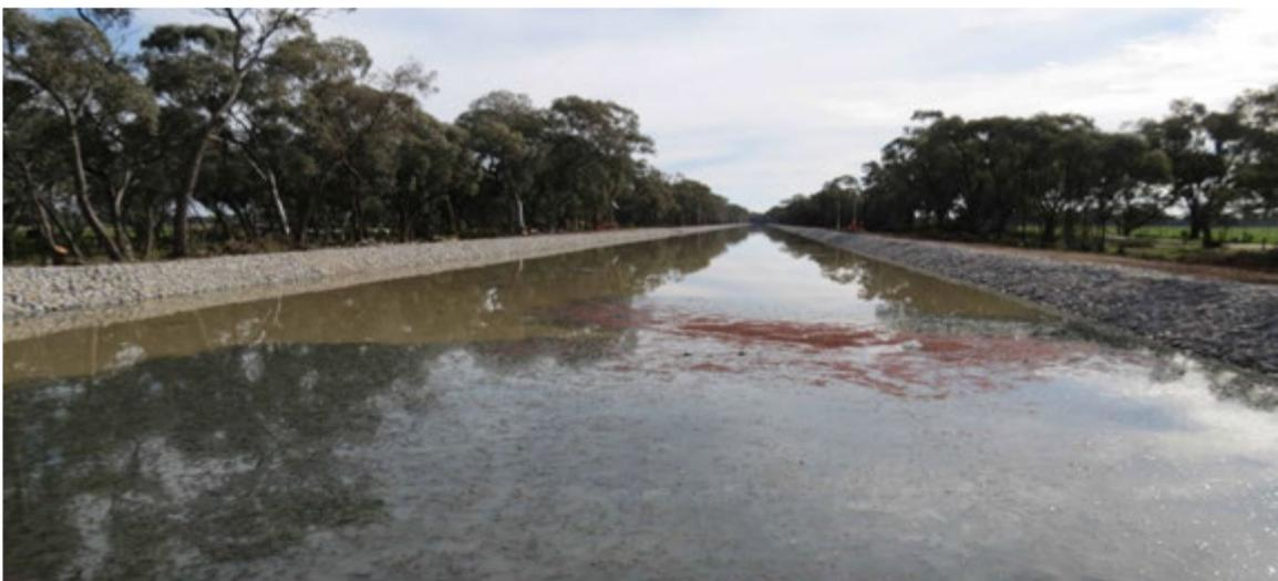
**Above: Channel 2/4/1 from the top-Clay lined, HDP lined, crushed rock and Rock wall finish. Works completed between May and August 2017.**
