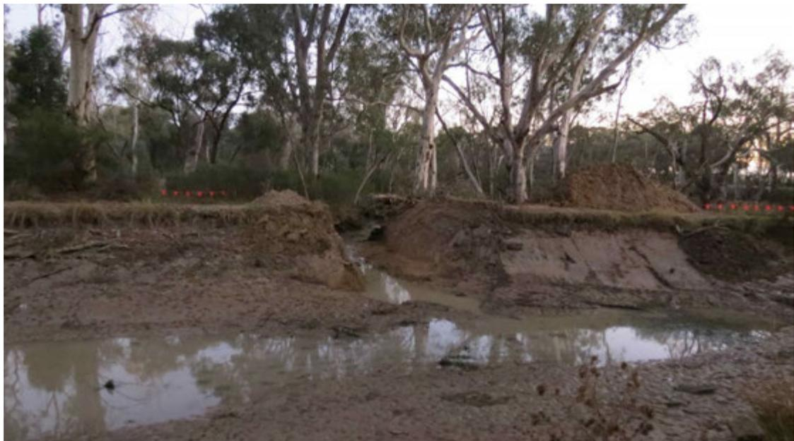
**Above: Channel 2/4/1 -cut made by excavator to drain water from the channel for works to begin.**
