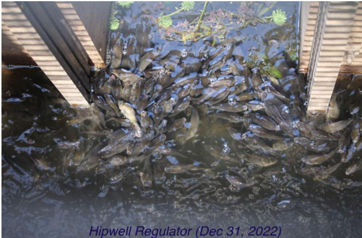
At 7:00am and 7:00pm the exit and entry gates on the fish lock operated to allow the fish (carp) on the forest side of the regulator to enter Gunbower Creek.
