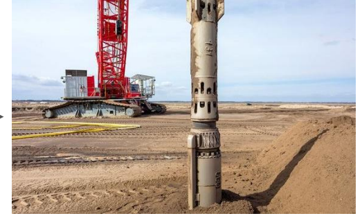
Preparation – compacting
