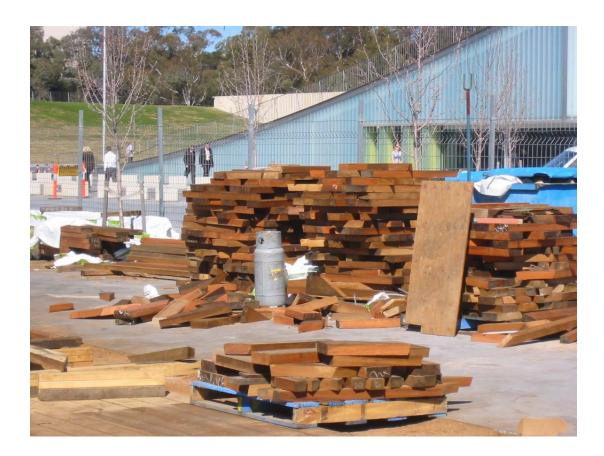
This is an example of avoidable timber waste created on site through a lack of understanding during specification. There will be a cost associated with its removal as well as the implications for life cycle analysis.
