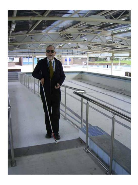
Salisbury Swimming Centre access upgrade including modification of male and female changerooms, building a unisex accessible change/toilet space, and installing a concrete ramp after widening the 25m pool. Total Cost \$
