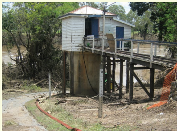
Gayndah Water Intake Plant damaged in 2011 – $1.2 million in restoration funds were required to replace the plant to pre-disaster condition.
