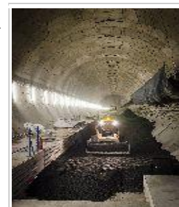
Inside Legacy Way in Brisbane, where tunnel backfilling is underway.
