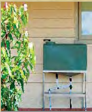
The Greywater Gardener 230, permanent greywater diversion and irrigation system.
